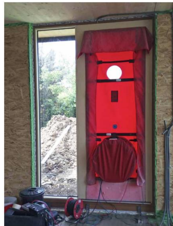
Blower-Door-Test | © BURIAN & KRAM Bauphysik GmbH
