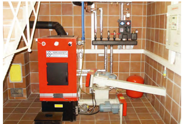
Hackgutkessel | © Tag-Putz
